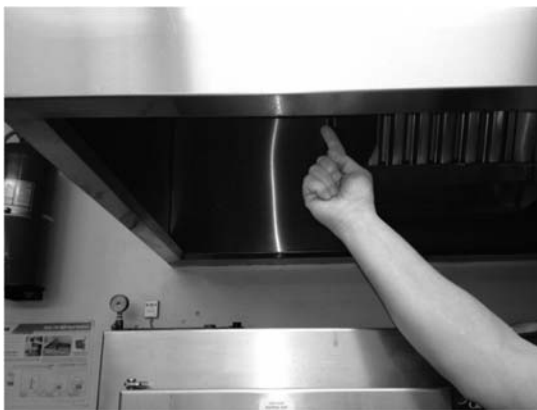
Look up under the hood to inspect for grease
