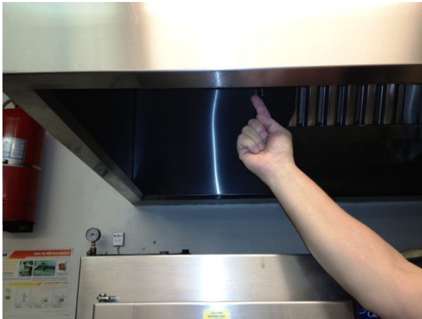
Look up under the hood to inspect for grease
